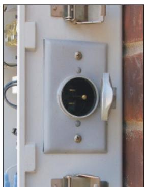
Connect the extension cord from the generator to the receptacle on the side of the panel, and start the generator. Then switch the MAIN/OFF/GEN switch to the GEN position. If the tank is full, the alarm and light will come on. Press the lighted button to reset the alarm, and the pump will pump the tank down to the normal level.
